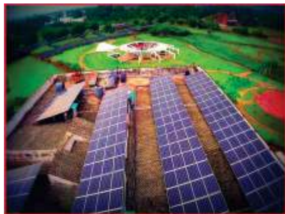
200 Kw Rooftop SPV Power Plant at Post Graduation College for Girls, Sec 42
