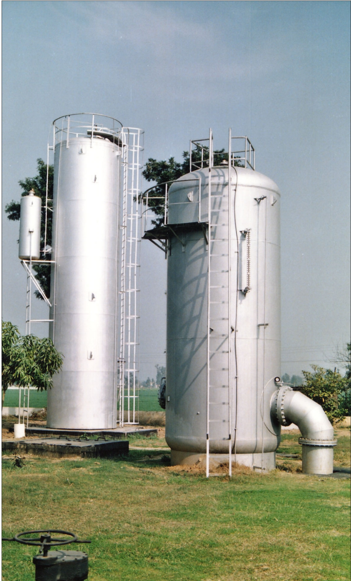
SURGE CONTROL EQUIPMENT AT WATER WORKS KAJAULI
