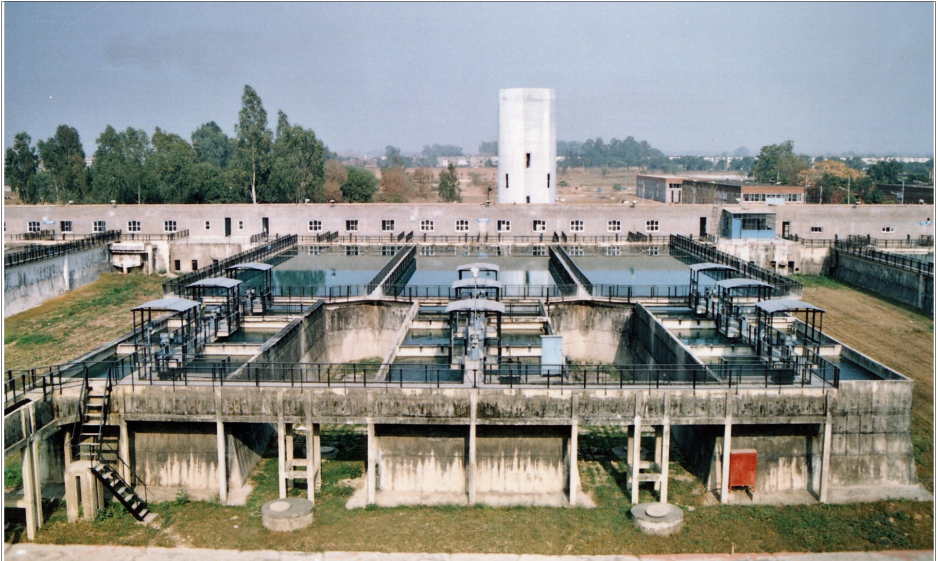
RAPID SAND FILTRATION PLANT AT WATER WORKS SECTOR 39, CHD
